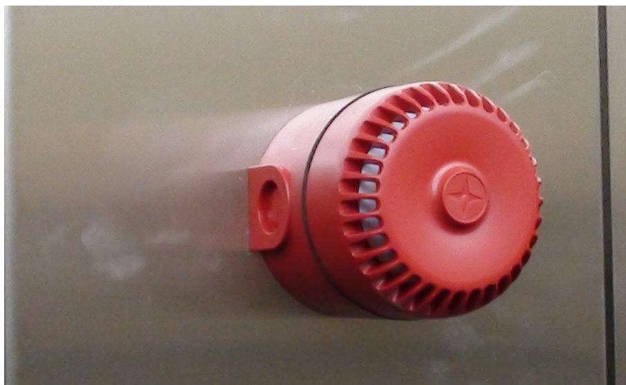
Figure 159: Signal horn on the valve manifold
